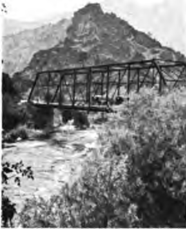
Klamath River bridge.
